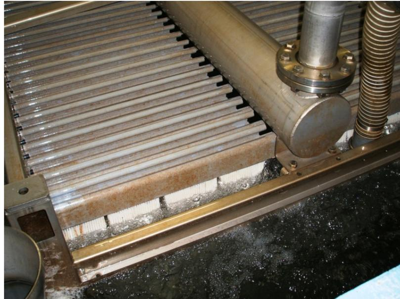
Picture 2: Filtration tank with submerged membranes
