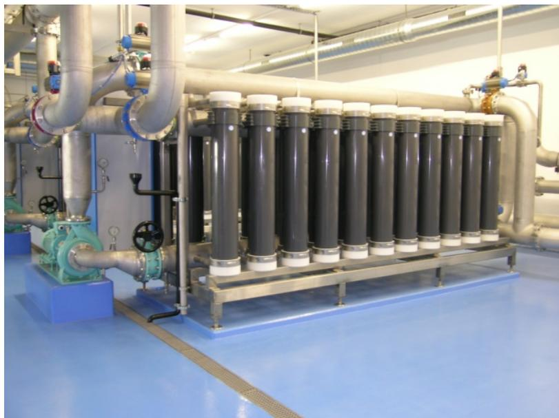
Picture 1: Membrane line with 41 pressure membrane modules
