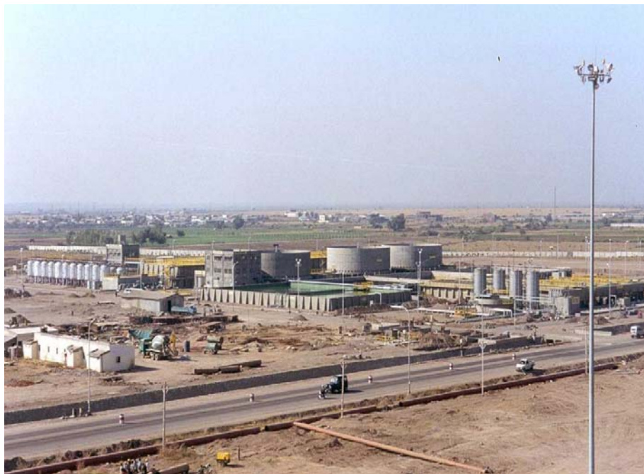
Fig. 1: Jamnagar Wastewater Reclamation Plant
