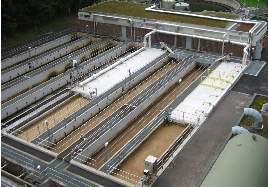
Figure 1: Membrane bioreactor plant Wädenswil, Switzerland
