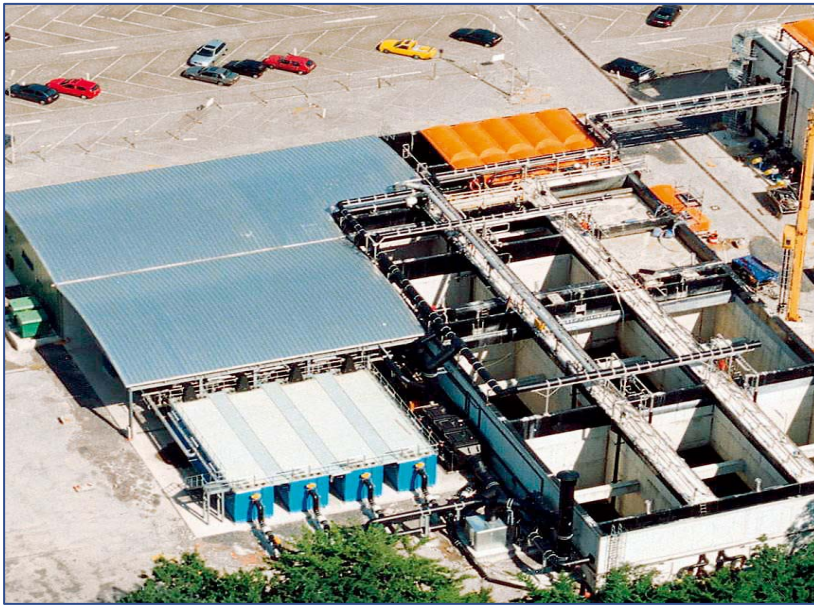
Fig.3 Schering MBR – Aerial View
