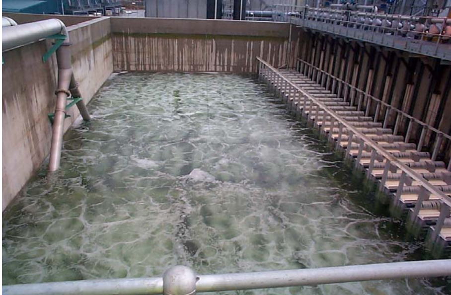
Fig.1 Daldowie MBR – Nitrification Process Step
