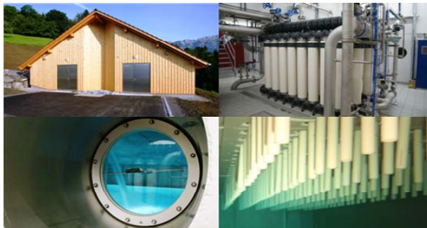
GRABS spring water treatment plant
